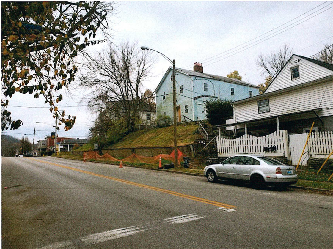
FIGURE 1 – TYPICAL VIEW OF 305 MAIN STREET
